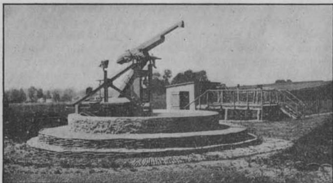
NO. 2.—FRENCH 75 MM. FIELD GUN ON FIXED MOUNTING FOR AERIAL DEFENSE OF PARIS.
